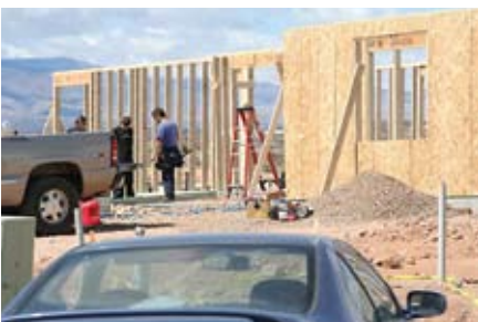
Construction of the Tunlii tribal housing development
