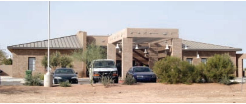
Revenues from gaming helped construct a new Elderly Center for members of the Ak-Chin Indian Community.
