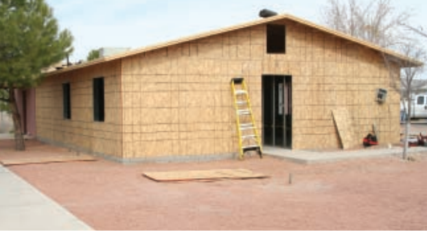
Left: A new home under construction on the Yavapai Apache Nation, one of 35 built in 2006.
