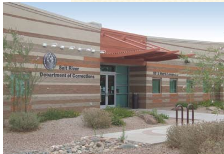
The new correctional facility at Salt River Pima-Maricopa Indian Community focuses on rehabilitation and includes a Boys & Girls Club on site to provide classes for detainees.
