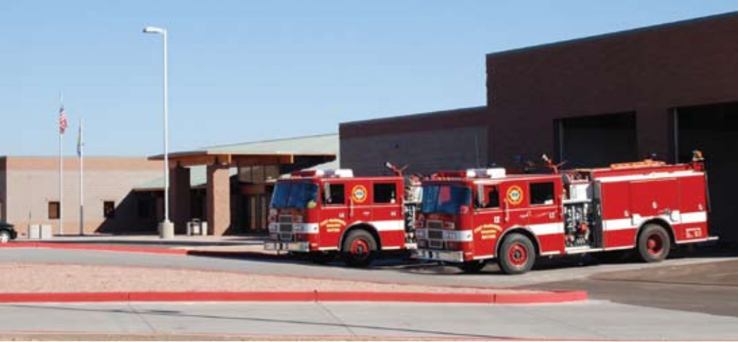
Nationally, according to the National Indian Gaming Association, tribes spend approximately 17% of their income to provide police and fire protection which benefits tribal members and their neighboring communities. Pictured is the new Justice Center at the Fort McDowell Yavapai Nation which was funded in part by gaming revenues.
